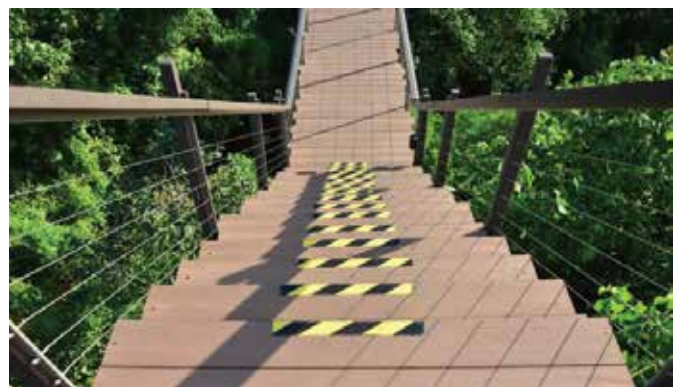
Anti-slip tape for stair.
